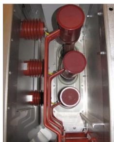
Gambar 2. Busbar Compartment
